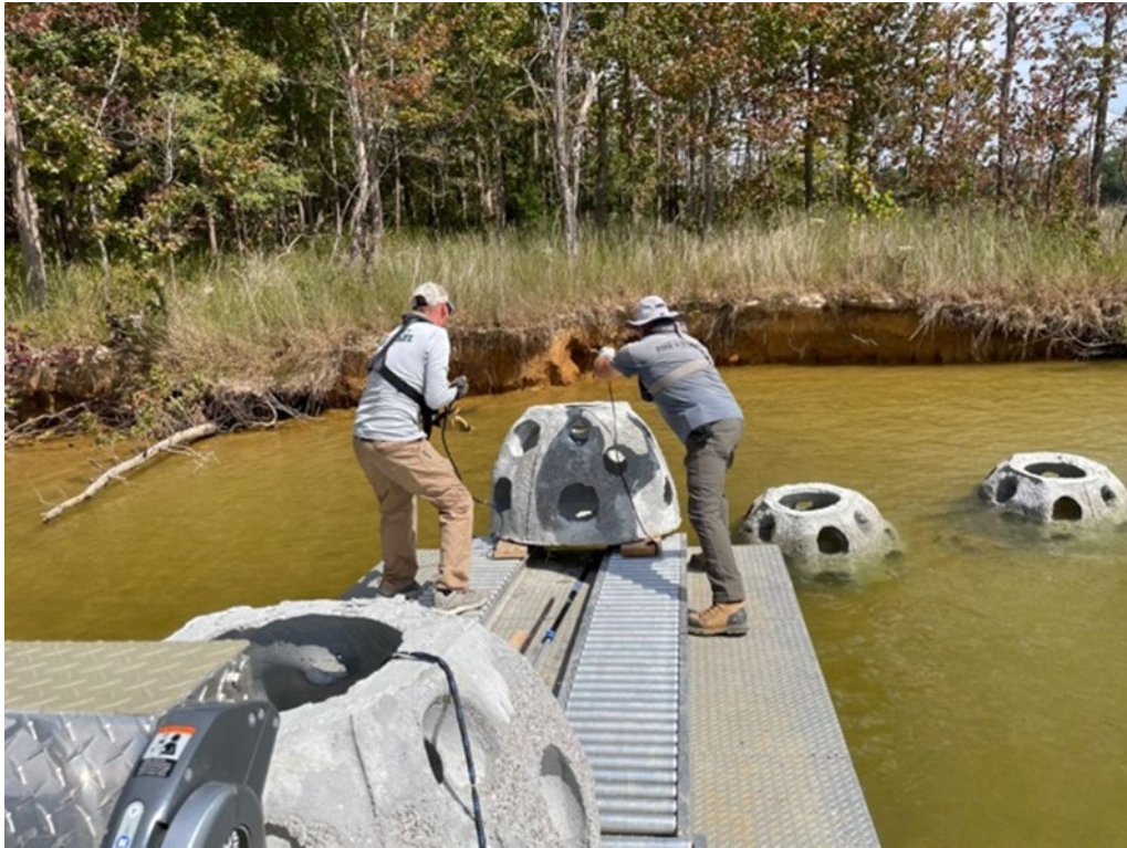
KDFWR staff installing a reef ball from their habitat barge.
